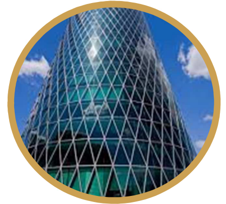
Westhafen Tower, Frankfurt
